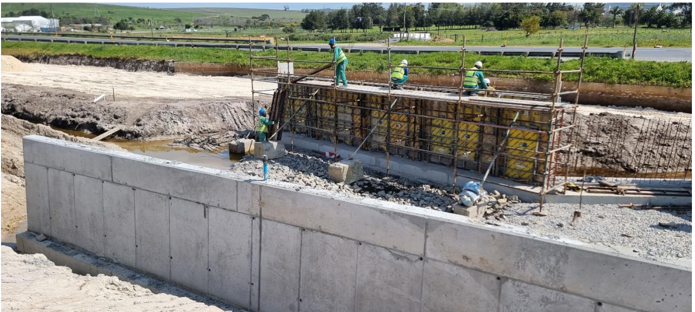
Sanddrift retaining walls
